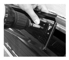
Secure PTAC unit to the bottom side of fan guard screen. When reattaching fan guard screen check for fan blade clearance.
