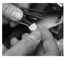
6. Using supplied wire nuts, attach wires from cell to wires from ballast. Matching blue to blue and red to red.
